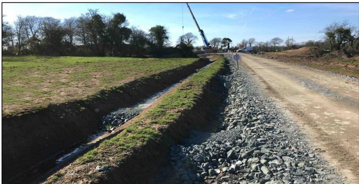
Figure 5-2: Separation of clean and dirty water drainage on wind farm site
